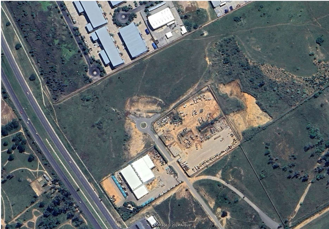
Figure 14: Existing access positions
