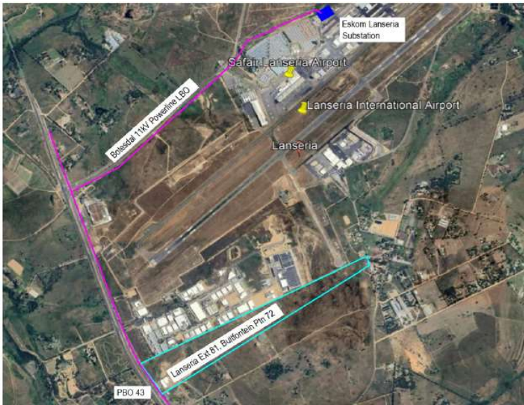
Figure 4: Existing Eskom Botesdal 11kV overhead line
