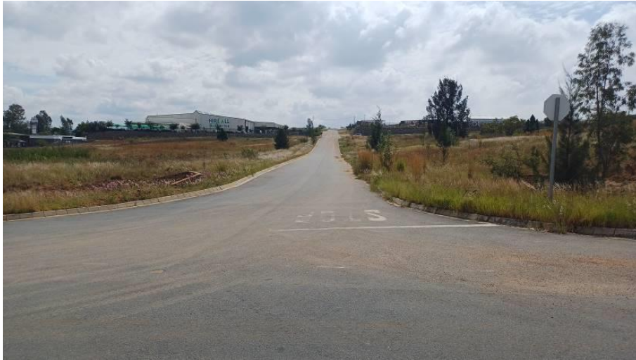
Township access road
