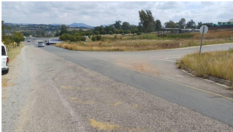
Intersection Boeing Street and township access road
