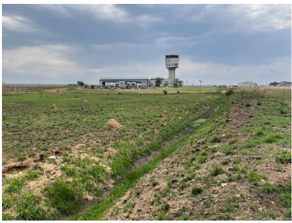
Photo 4. Constructed stormwater drain
