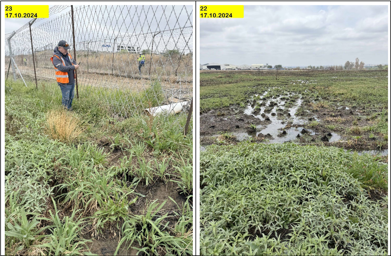
Photo 5. Storm water drains along the southern boundary
