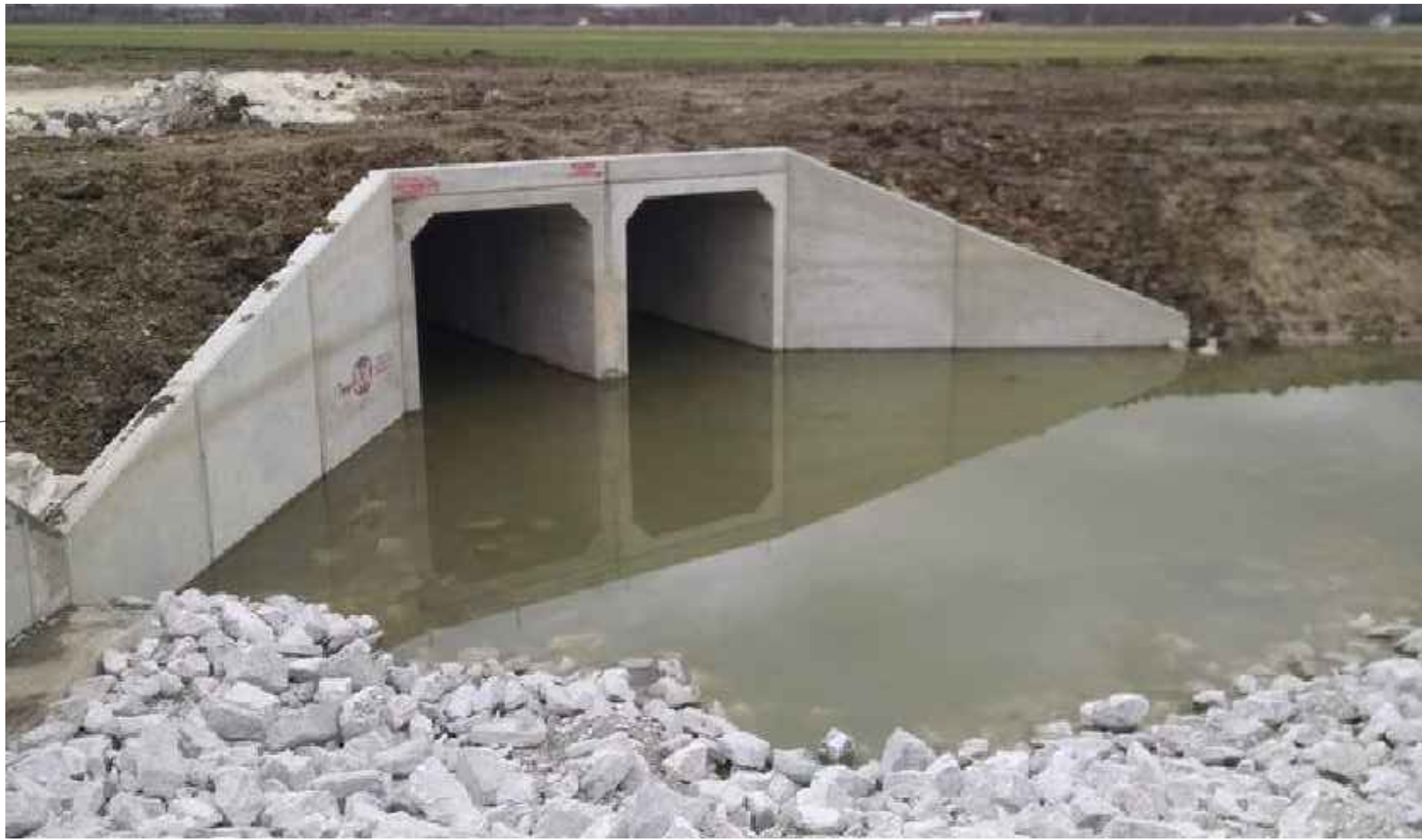
TYPICAL CULVERT OUTLET STRUCTURE TO NATURAL WATER COURSE
