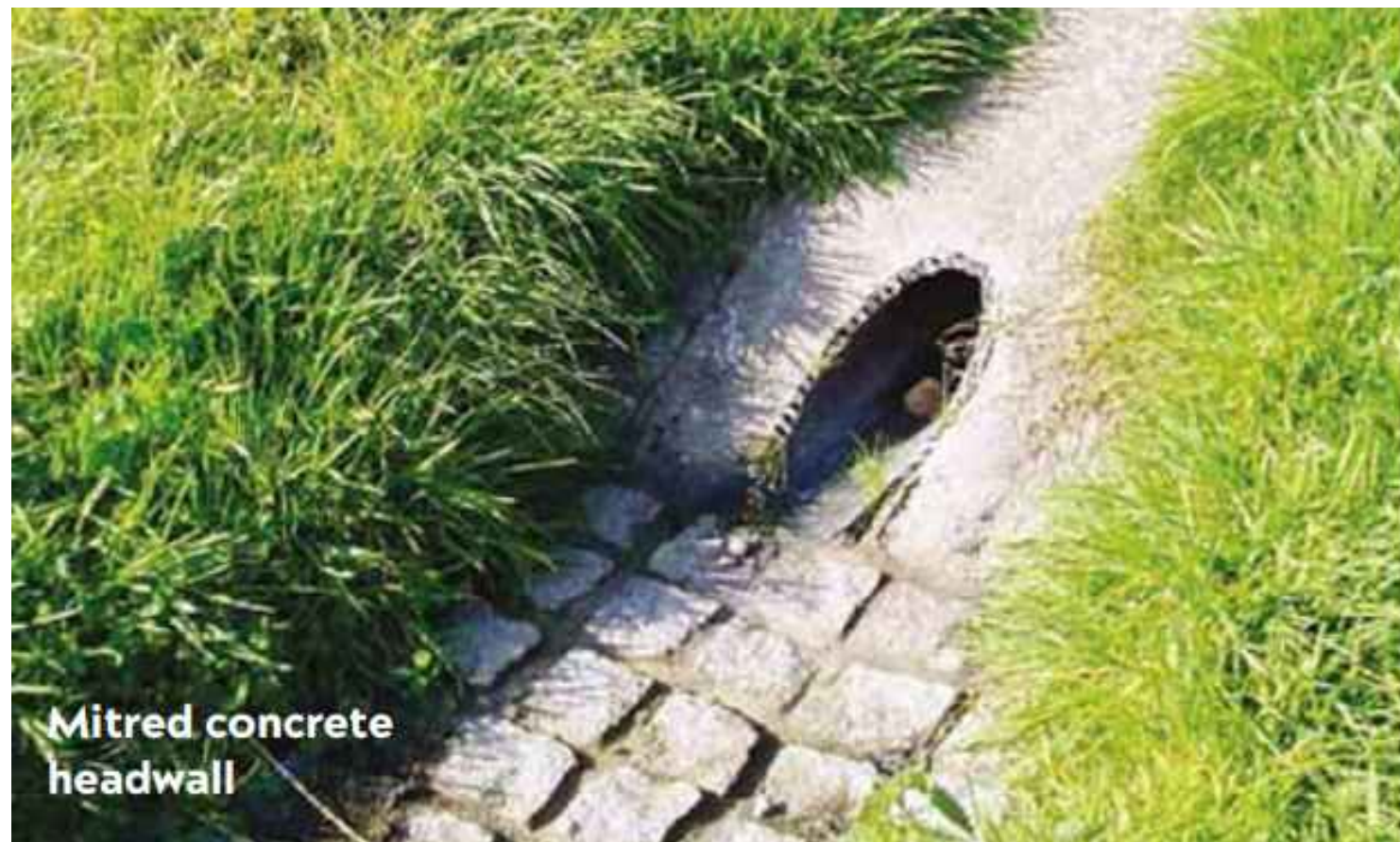
SUBSOIL OUTLET TO RECONSTRUCTED WETLANDS
