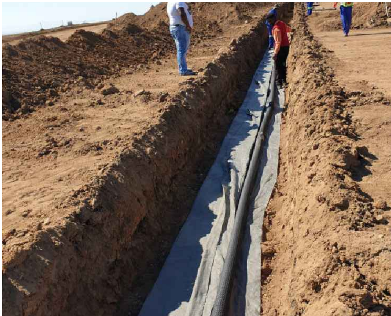
SUBSOIL PIPE SYSTEM
